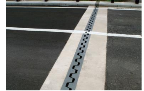
⑤ HYBRID sheet for preventing the peeling off
