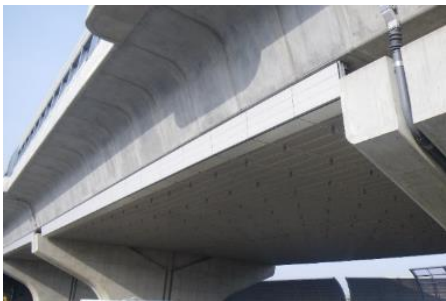
Prevention device for bridge fall③
